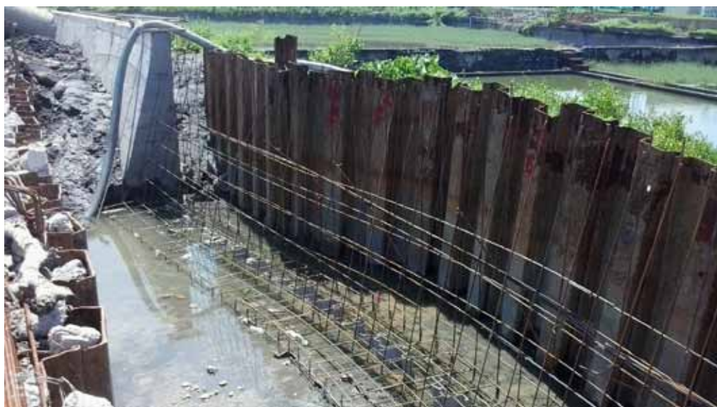
Pingtung Rope ditch recon- struction project
