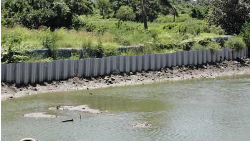
Kaohsiung Black Bridge drainage improvement project
